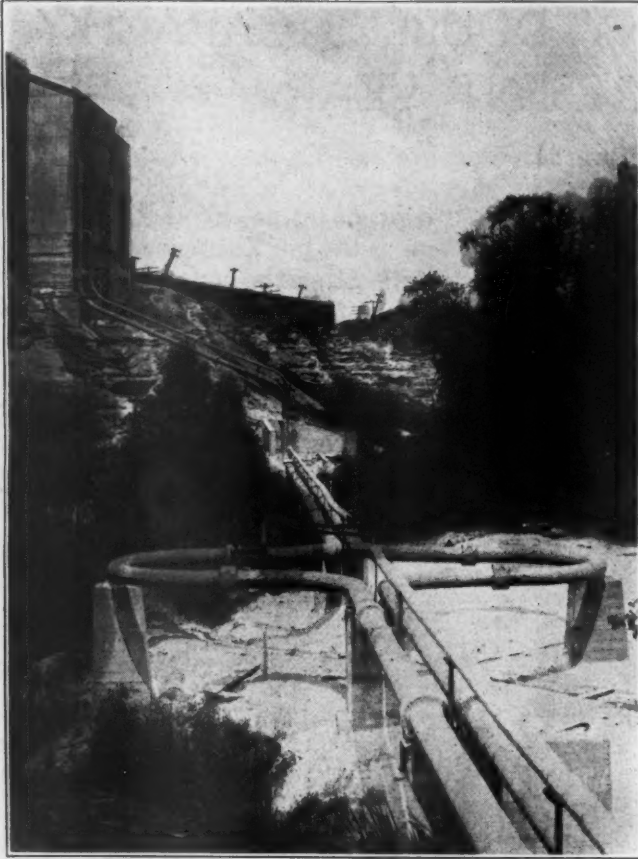
Close-up of Steam Pipes Showing Expansion Bends
